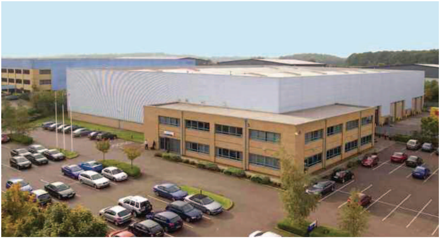
Meridian Business Park - New Acquisition January 2007
